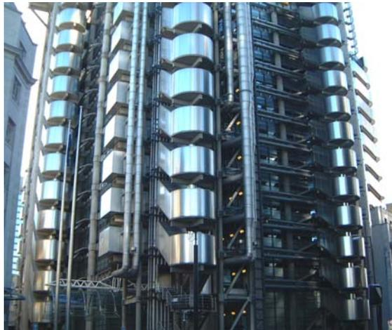
**Figure 3:** Services and stairs located on the exterior of the Lloyds Building in London
