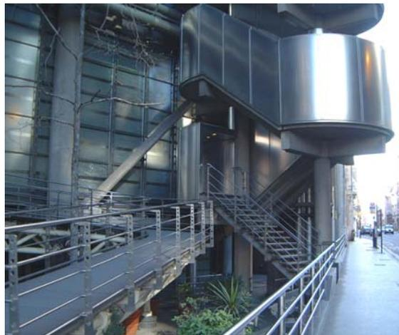
**Figure 4:** Stainless steel cladding, handrails and balustrade systems (Lloyds Building, London)
