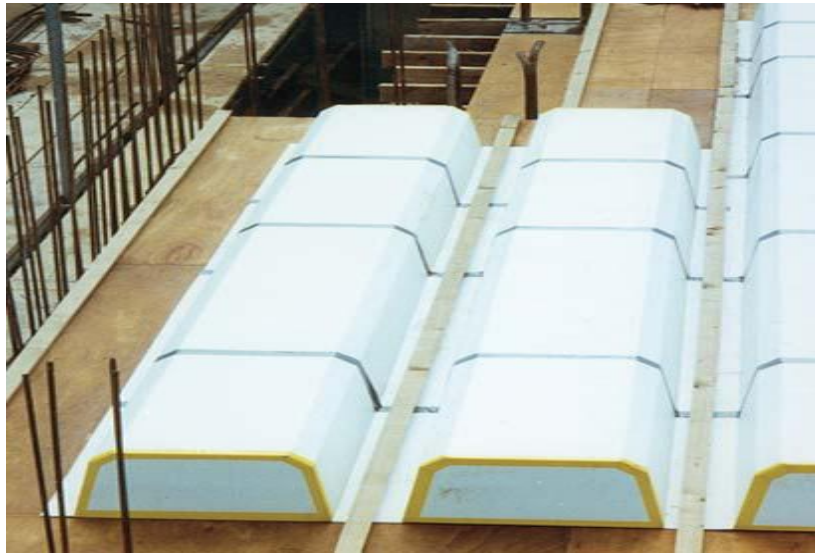
Figure 2.2. EPS Trough mould (Cordek, 2009c)
