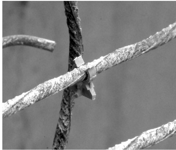
Figure 2.10 A-shaped spacer still attached to reinforcement with no sign of corrosion after 36 years of use in car park.[Shaw, 2008]
