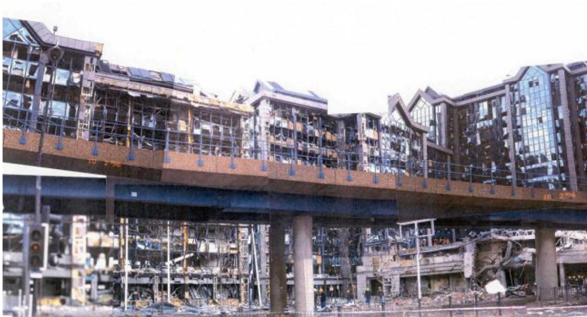
Figure 1-1: Effect of an explosion on office buildings in London's Docklands area.
