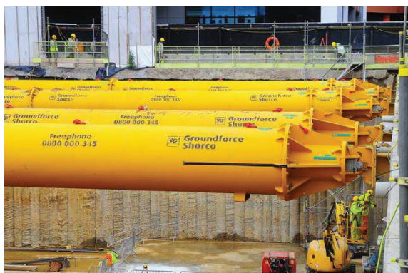
(a) End part of huge hydraulic props
