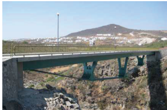
(b) San Miguelito creek footbridge, Mexico (Madrazo-Aguirre et al. , 2015)
