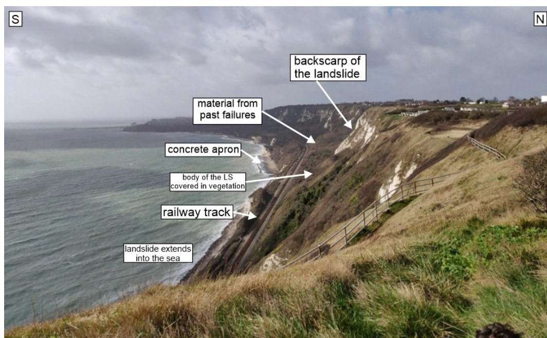
Figure 5.3. Folkestone Warren landslide (viewed from the eastern end) with chalk backscarp and railway track visible, linking Folkestone and Dover.
