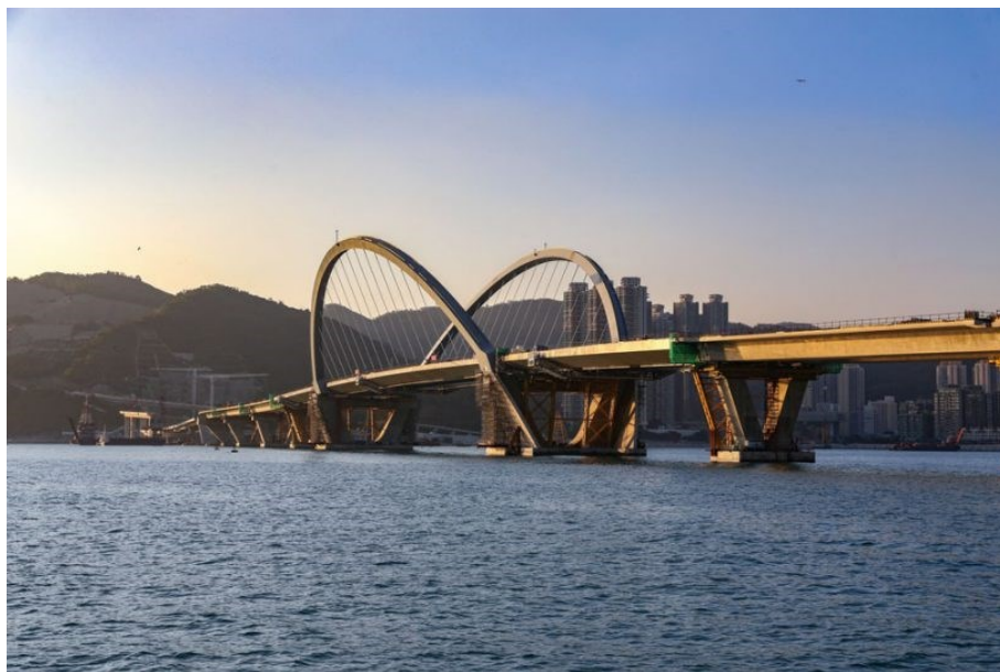
Figure 1.2: The Tseung Kwan O Cross-Bay Link Bridge, Hong Kong, China ( https://www.constructionplusasia.com/hk/cross-bay-link-tseung-kwan-o/ )
