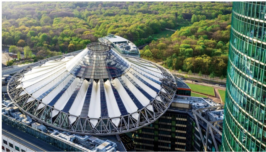
Figure 1.1: The Sony Centre, Berlin, Germany ( https://www.arup.com/projects/sony-centre )
