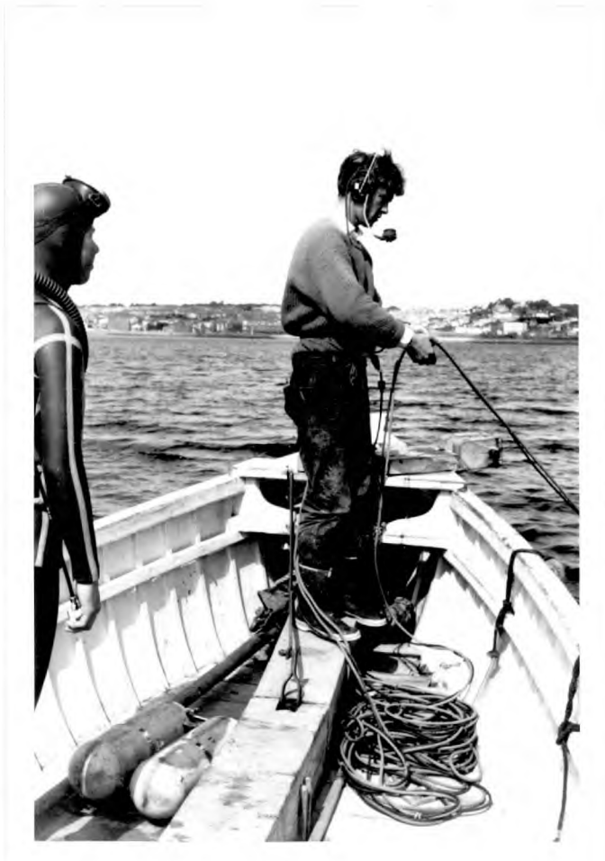
Figure 6. The "surface control" using underwater telephone.
