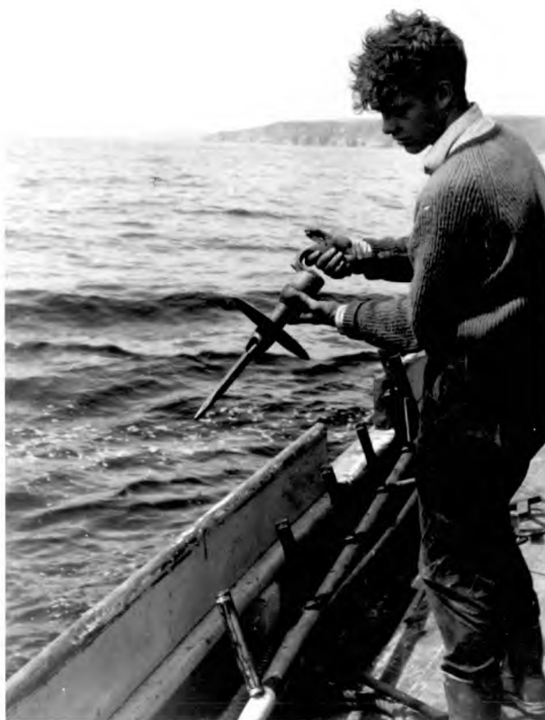
Figure 12. The compressed air operated percussion hammer.
