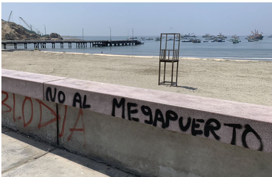
Figure 1. A wall on the boardwalk displays the message “No to the megaport.” In the background, you can see the beach, the artisanal fishing pier, and the sea dotted with artisanal fishing boats. To the far left, cranes are visible, working on the construction of the megaport.
