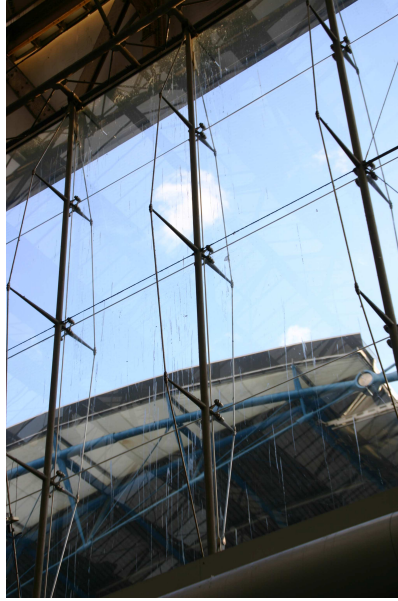
(b) London Waterloo Station, UK
