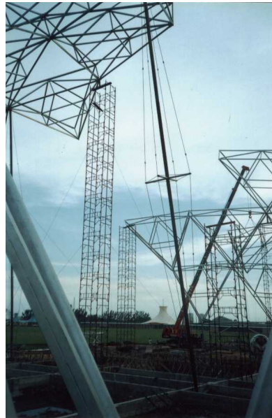
Figure 1.2: The single-bay prestressed stayed column used as the temporary support during the construction of the Rock in Rio III stadium (Andrade et al. , 2003a; Andrade et al. , 2003b).
