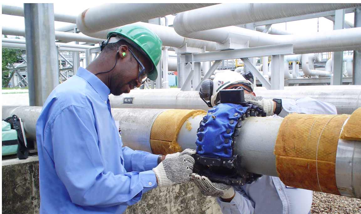
Figure 1.1: Guided wave screening of an insulated pipeline [1].
