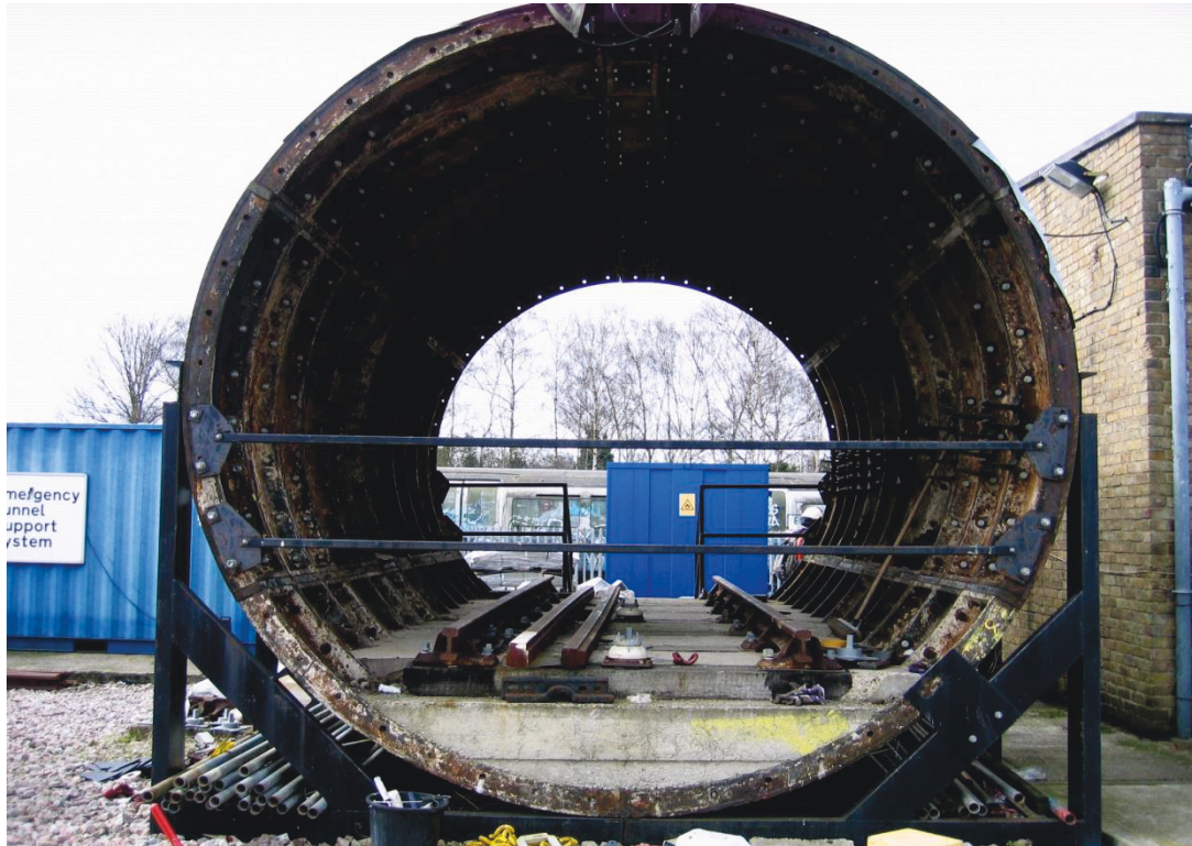
Figure 3-1. A section of GCI tunnel constructed above ground at the LU Acton Depot.
