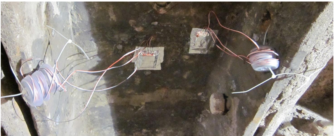
Figure 3-11. Strain gauges on segment 2.
