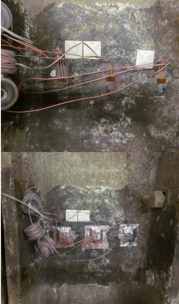
Figure 3-10. Strain gauges on segment 1. Without protective coating (left) and with protective coating (right).
