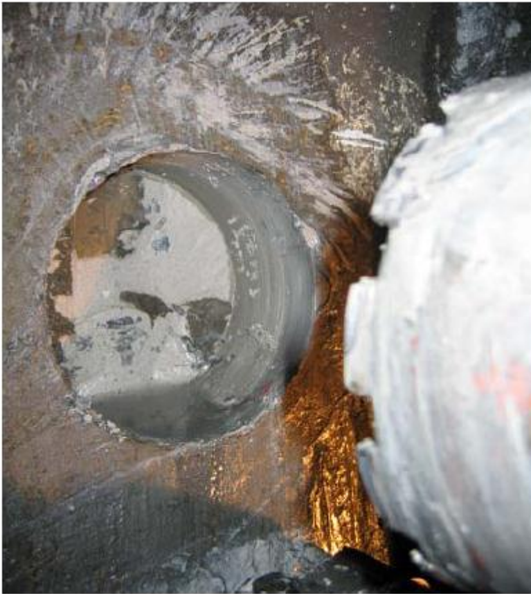
Figure A-12. Instrumented portion of skin removed from tunnel segment (Tube Lines, 2006).
