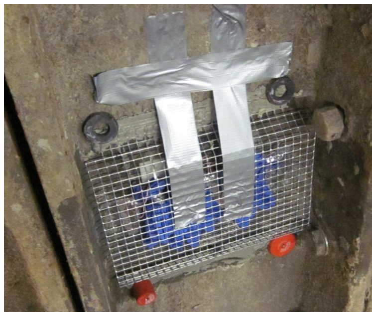
Figure 3-13. Wire bracket to protect strain gauge rosettes.
