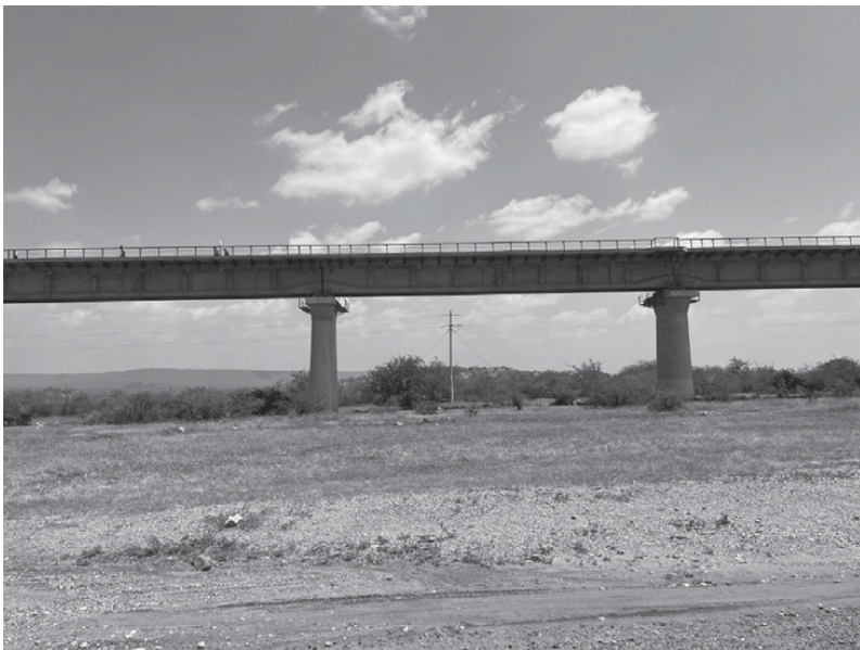
Figure 0.9: The Export-Import Bank of China-funded standard gauge railway in Kenya
