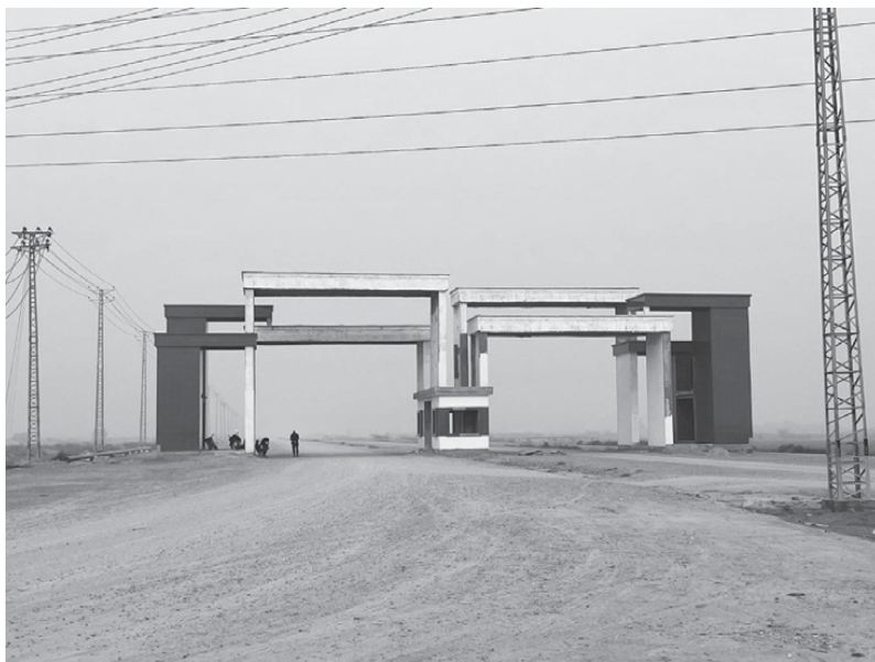
Figure 0.1: Gates to the Allama Iqbal Industrial City Special Economic Zone in Pakistan, under construction
