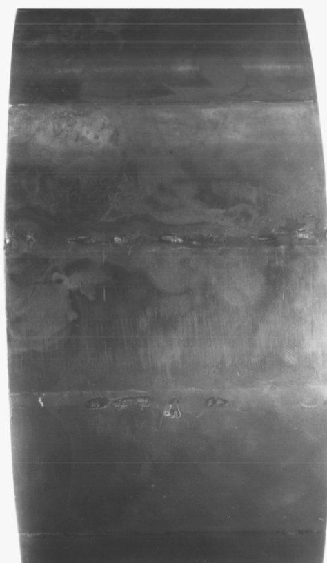
upper figure 2.16. Closing tee-butt weld viewed from inside.
