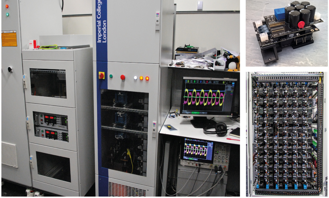
Fig. 5: Experimental Setup. Left: Lab-Scale multilevel converter demonstrator with external power supplies. Top Right: SM design with switchable SM capacitor. Bottom Right: Array of 60 SMs arranged into 6 stacks, director switch for operation as AAC at the bottom of each stack.
