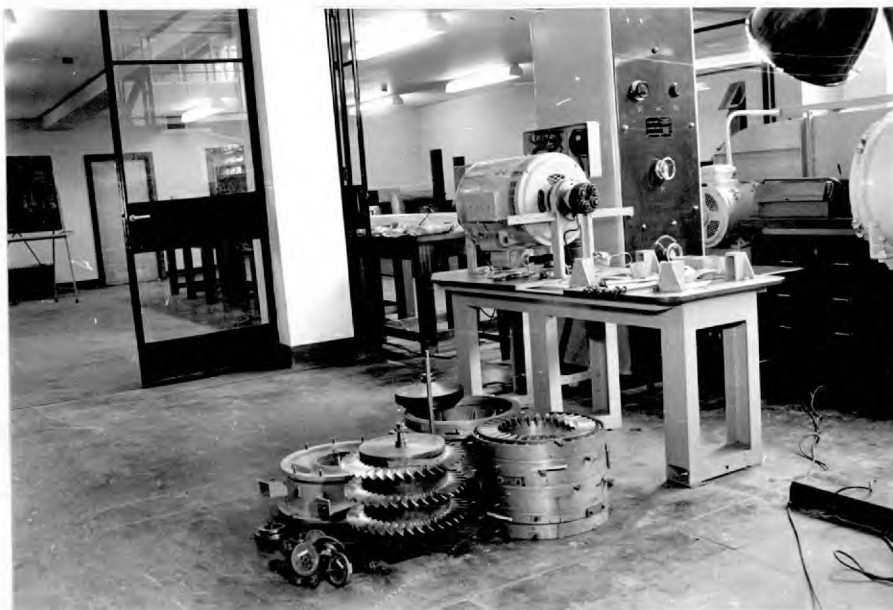
Components of the Compressor with the Motor on the Foundations
