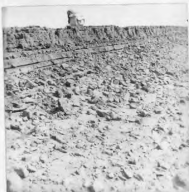
PLATE 60. ANGULAR MUD BLOCKS ON SIDE OF CREEK CHANNEL.
