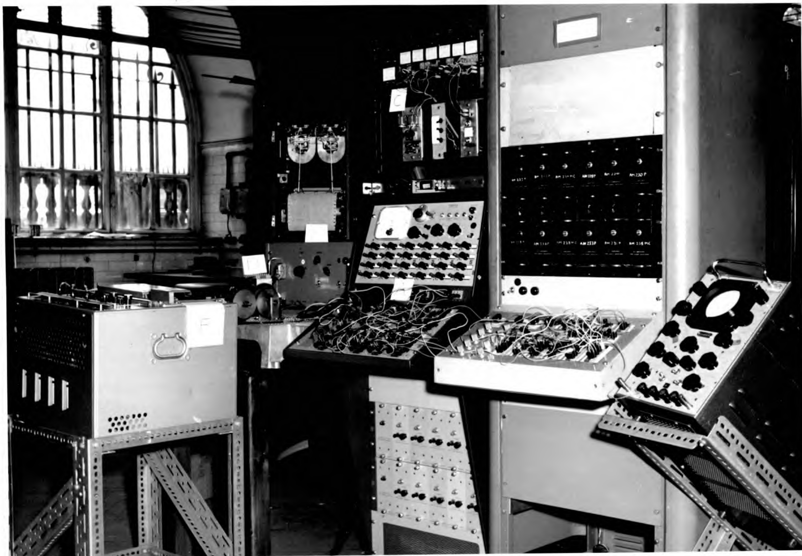
FIG. 10. ANALOGUE COMPUTATION EQUIPMENT
