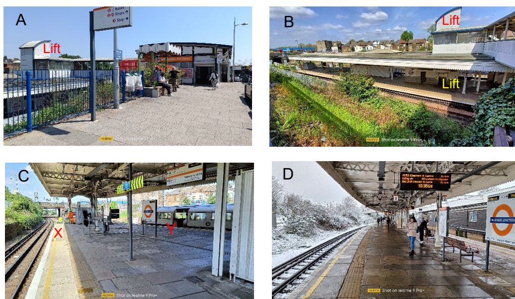
Figure 3.4 The station layout at Willesden Junction train station showing (A) the entrance to the station and access bridge across the railway tracks to the lift. (B) the lift from the station concourse to the platform, (C) the walk from the lift to the overground (X) and subway (Y) trains and (D) the subway track in the Elephant & Castle direction.
