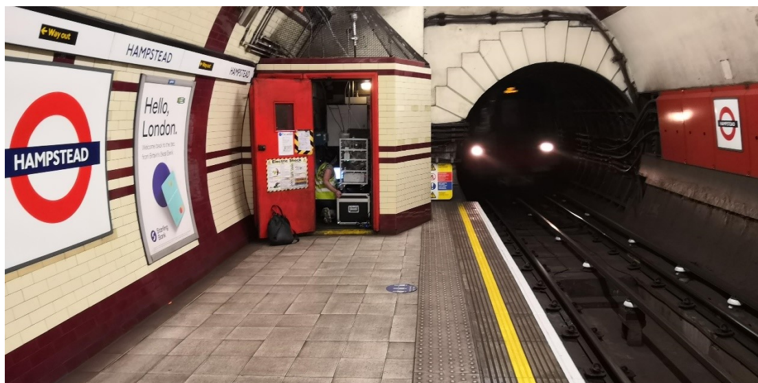
Figure 3.9: The Mobile Reference Station (MoRS) in the air quality facility on the northbound Hampstead subway platform being co-located alongside a Partisol 2025.
