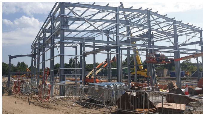
Figure 1.1: Newton Heath rail maintenance depot constructed as a single-span steel portal frame (NSC, 2020)
