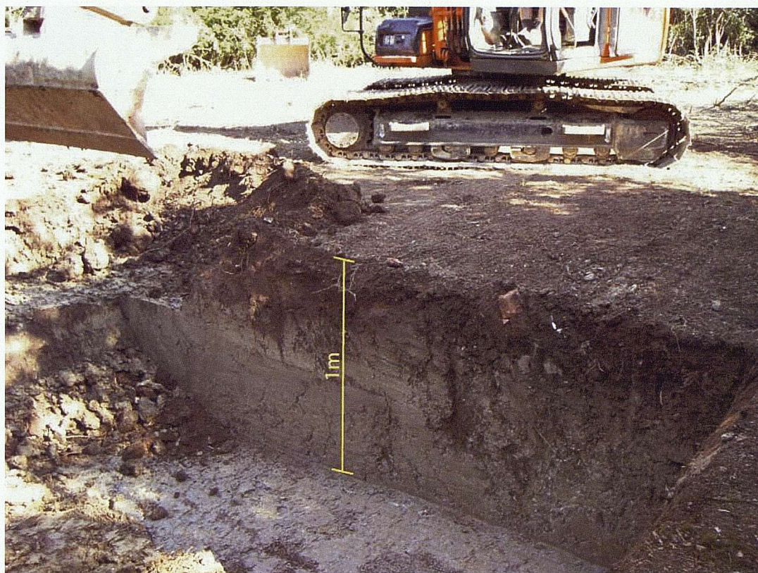
Figure 6.16 The initial stages of the excavation, 1m depth topsoil is 20-30cm thick going directly into the weathered top of the Gault Clay
