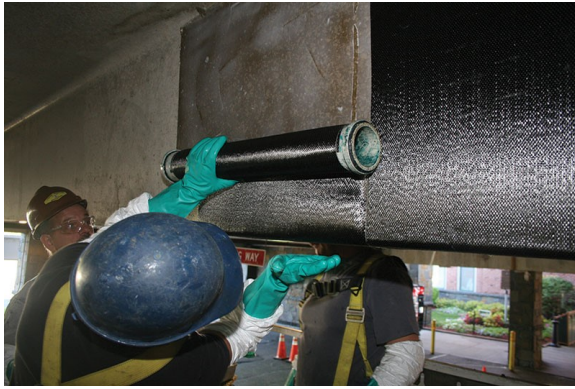
Installation of U-shaped jacket around beam
