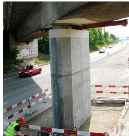
Bridge pier repaired with precast UHPC
