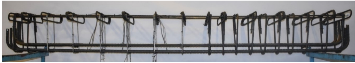
Assembled steel reinforcement cage of group 1 beam
