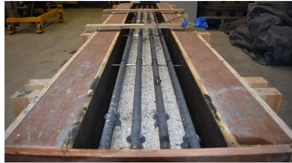
RC beam in mould
