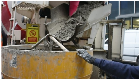
Ready-mix concrete loaded into concrete skip
