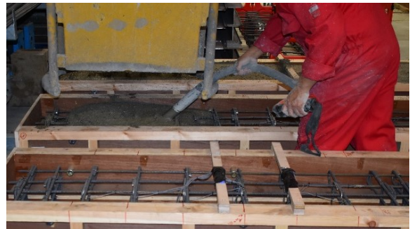
Pouring and vibrating concrete in mould
