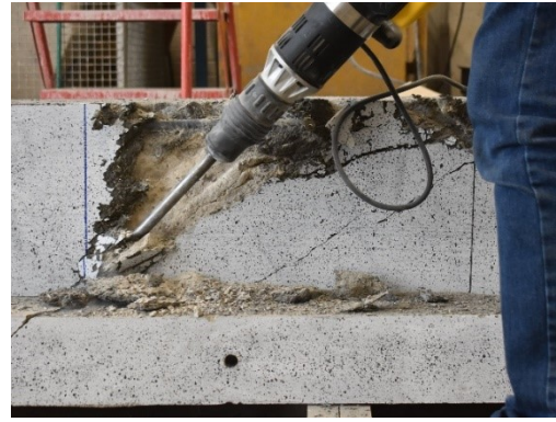
Intermediate phase of jacket removal
