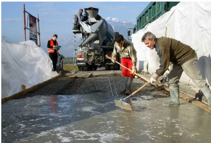
Bridge deck repaired with cast in-situ UHPC
