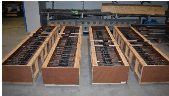
Placement of steel reinforcement cages in moulds
