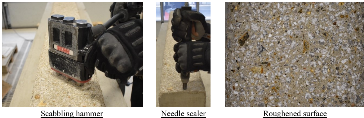
Figure 3.24 – Method for roughening bonding surfaces of RC beams
