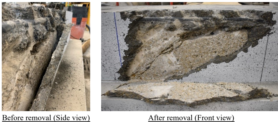
Figure 4.40 – Partial removal of UHPC jacket of specimen B6 (Front FOV)
