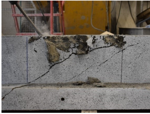
Initial phase of jacket removal
