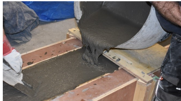
Casting UHPC from final position
