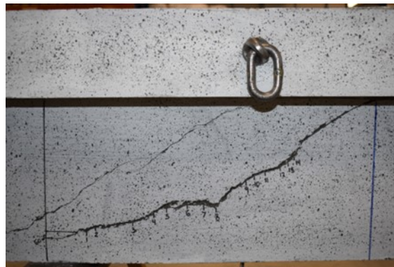
Measurement points on critical shear crack (Specimen B6 – Front FOV)
