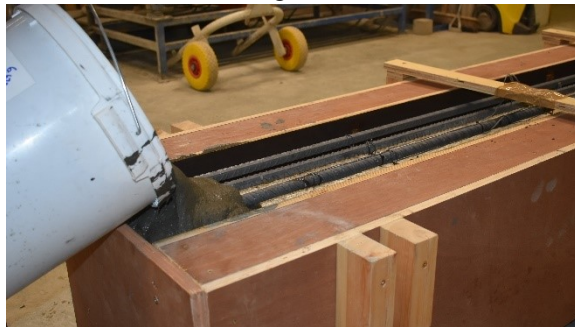
Casting UHPC from initial position
