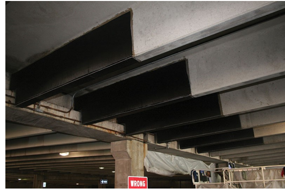
Installed U-shaped jackets
