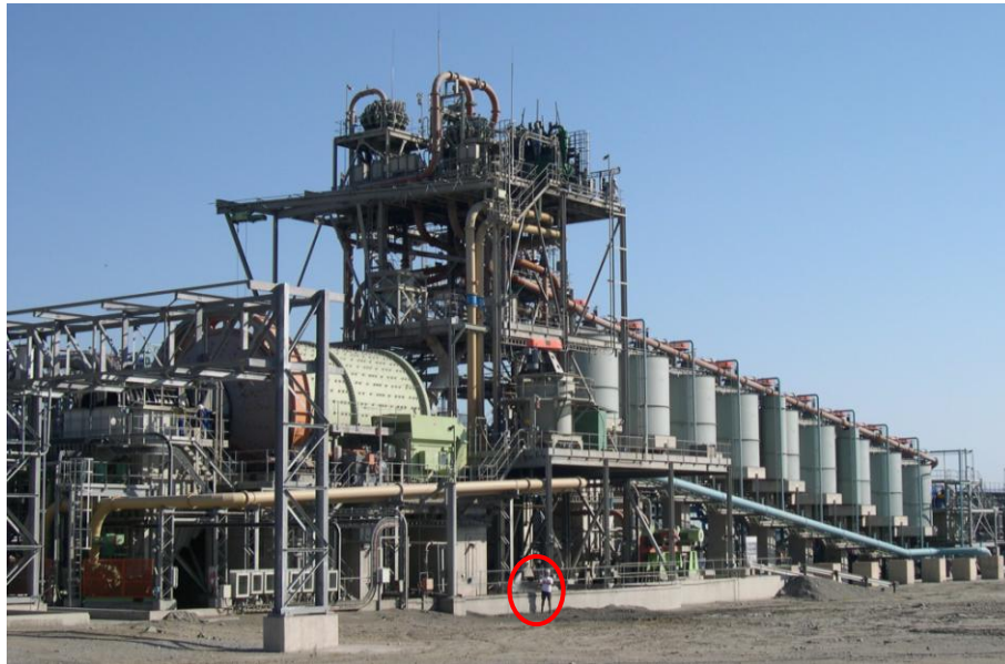
Figure 2-2. Bank of flotation tanks, Western Limb tailings retreatment plant. Ellipse highlights person for scale.
