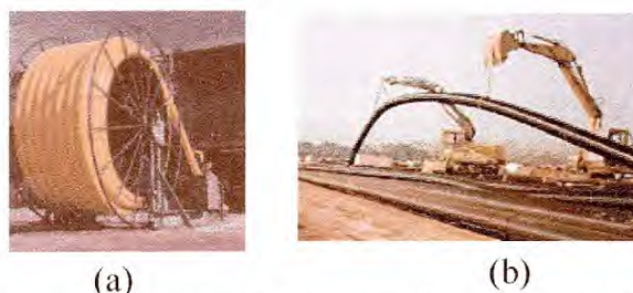
Figure 1.1 (a) Long lengths of pipe supplied in coil ( from http://www.wavin.co.uk ) (b) Laying of plastic pipelines ( from http://www.pe100plus.net )
