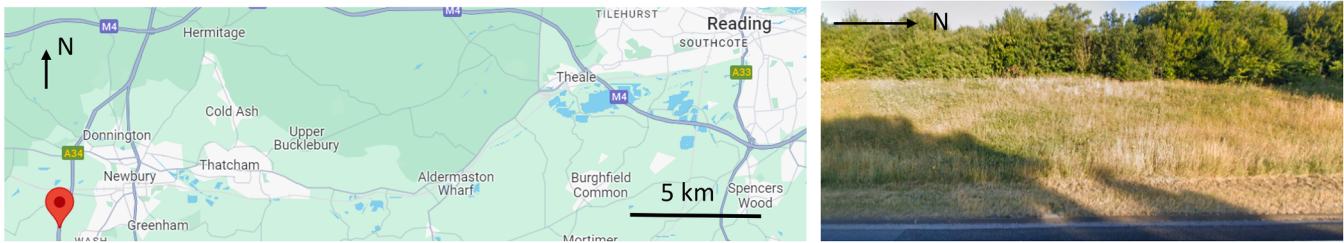
Fig. 1. Cut slope located in Newbury covered by grass and shrub.
