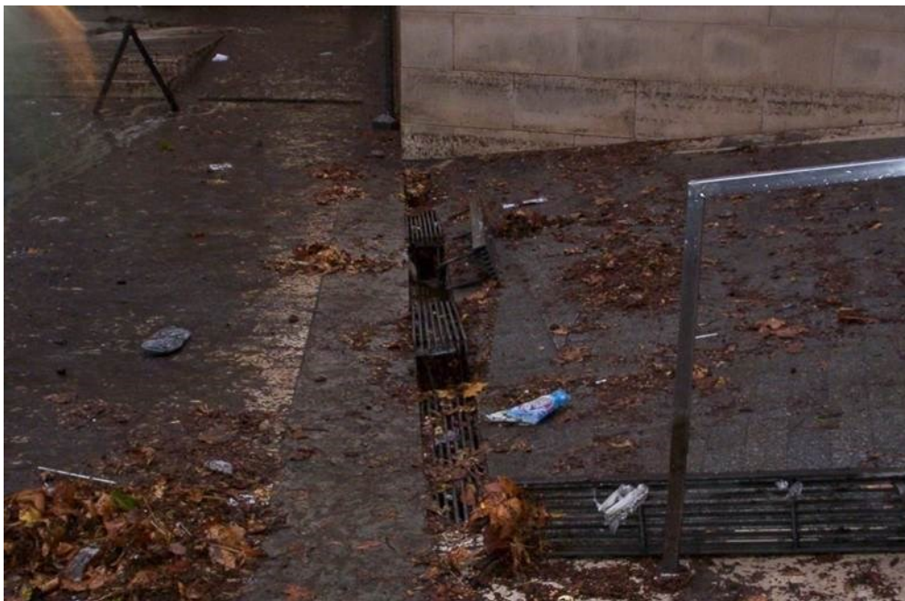
Figure 30. Flooding in Praça 8 de Maio caused by the rainfall event of 21 September 2008 (source: Diário de Coimbra ).
