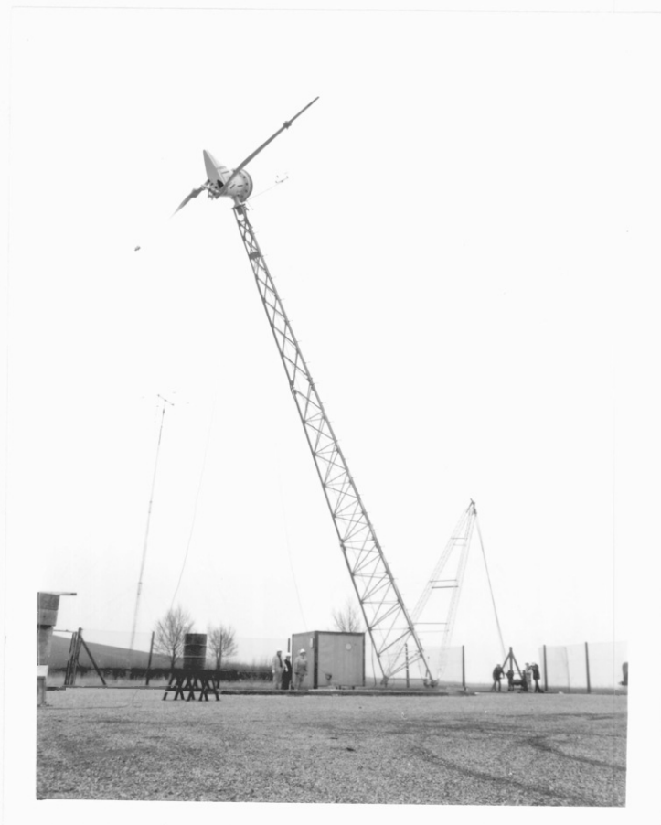
FIGURE 4.5 ERECTION OF L916 WECS (NOTE BOOM ANEMOMETER)
