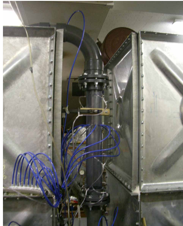
Fig. 9 Photograph of the siphon rig, showing the aerator
