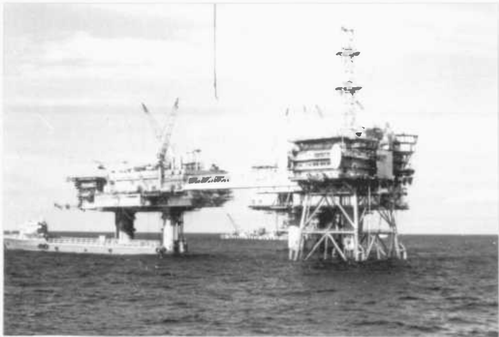
Plate 8 - Steel and Concrete Structures - Frigg Field
