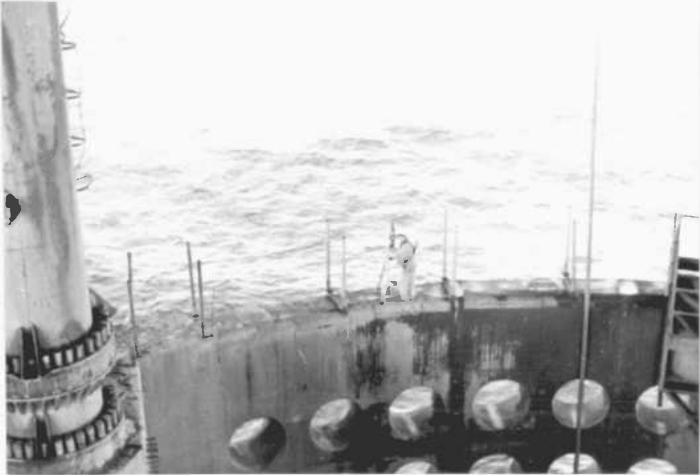
Plate 12 - View of Survey Station on Outer Concrete Wall of C.D.P.1.
