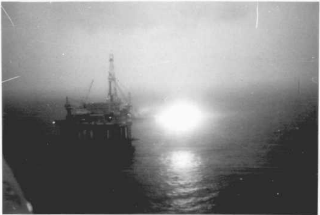
Plate 9 - Concrete Structure - C.D.P.1 - Frigg Field
