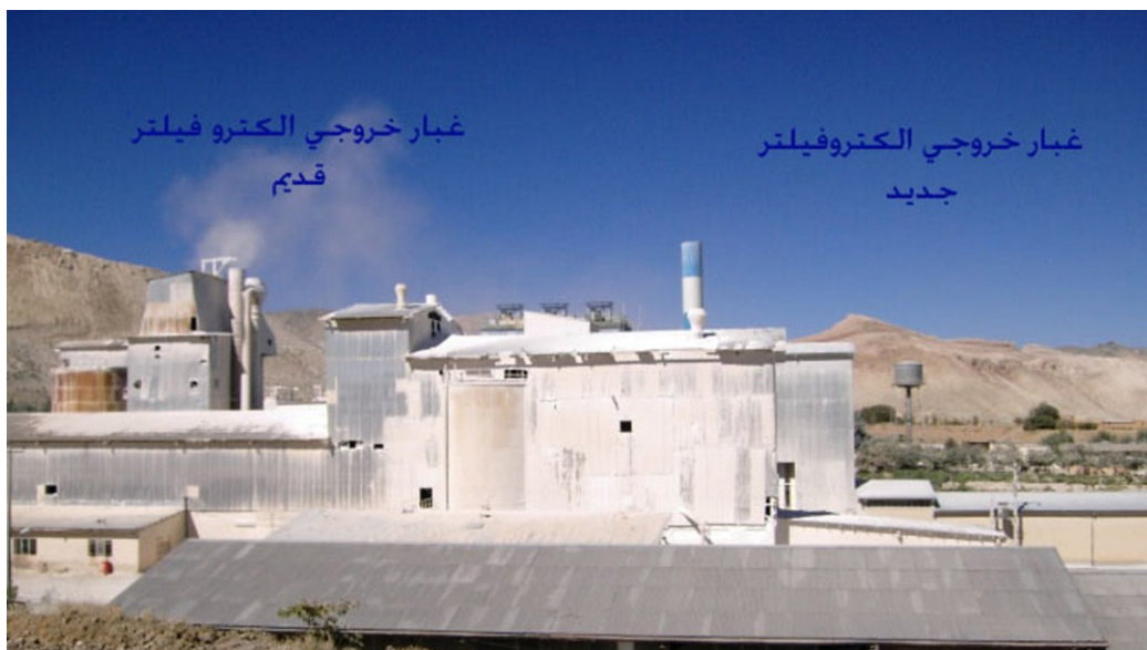
Figure 21: The difference between emission of air pollutants between the old (left) and the new (right) industrial electro filters at a gypsum manufacturing plant (Khorasan Gypsum, 2013)
