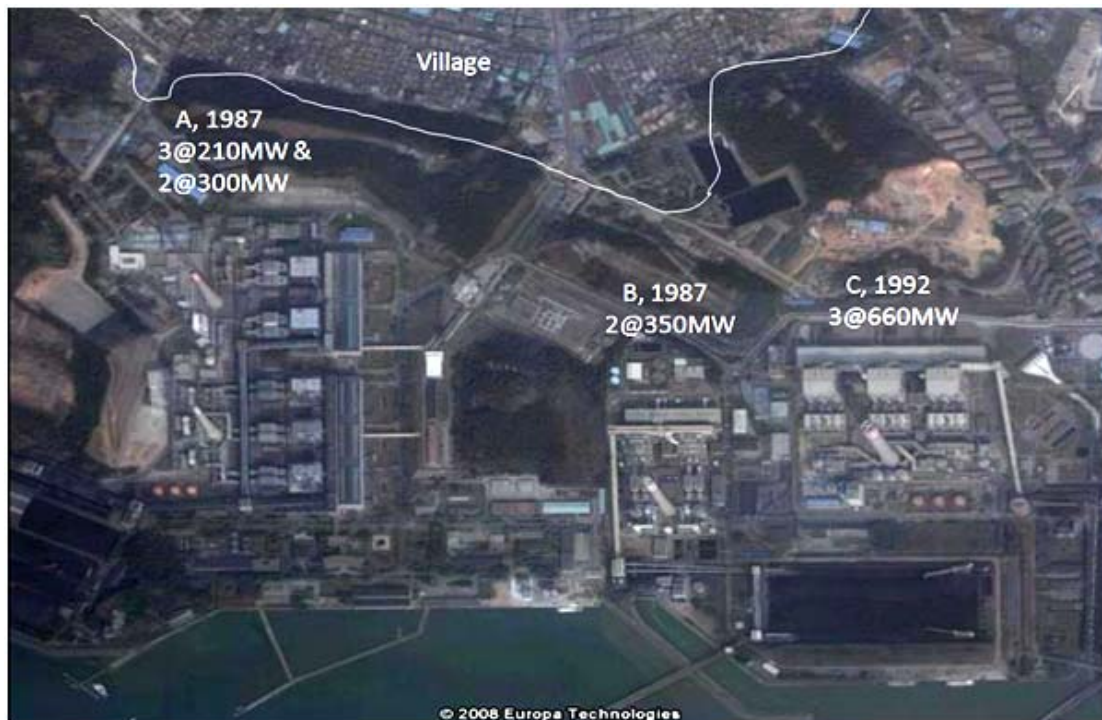
Figure 4-1 Shajiao ABC Plant, Guangdong, China
