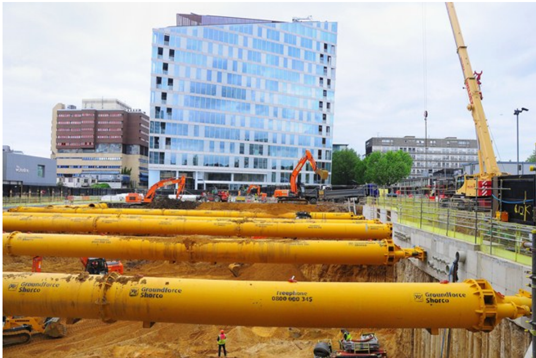
(b) Conventional 'super struts' as excavation props
