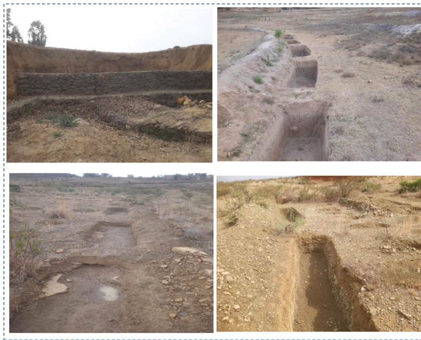
Fig. 7. Post-conflict soil and water conservation efforts in selected watersheds: (a) check dams in Atsbi, and (b) deep trenches in Atsbi, (c) Abergelle-Yechila, and (d) Samre.
