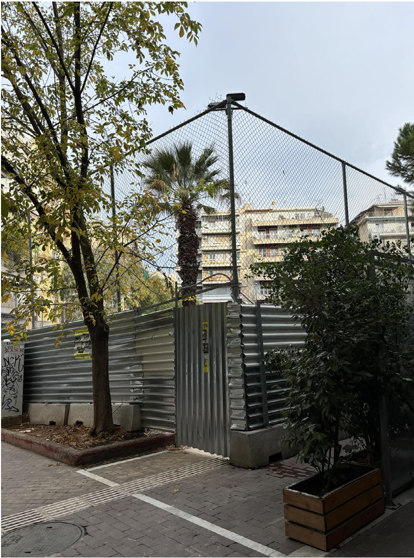
Figure 1: The entrance to the metro station construction site at Exarcheia Square (photo by Elia Apostolopoulou)
