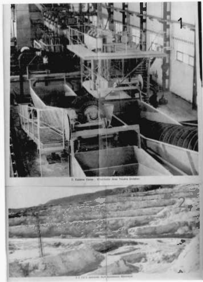
Fig. 2.5. Photographs of the Kirka operation: (1) the washery showing the spirals, hydrocyclones and scrubbers; (2) the open pit showing 3 m benches.
