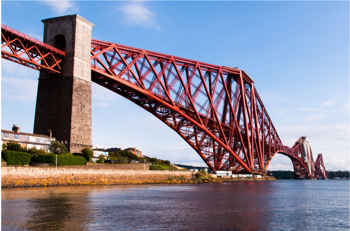
Figure 2.1: The Forth Bridge, Queensferry, Scotland with CHS main compression members.
