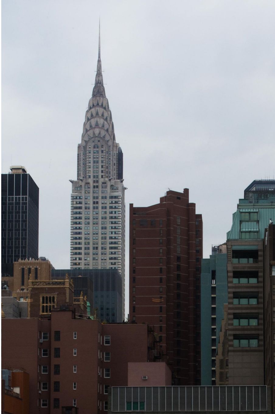
Figure 1.1: The Chrysler Building, New York with stainless steel cladding.
