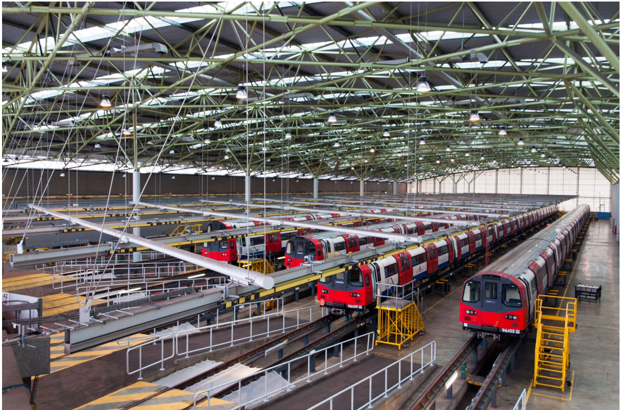
Figure 2.4: Stratford Market Depot, Newham, London with a CHS truss supported roof.
