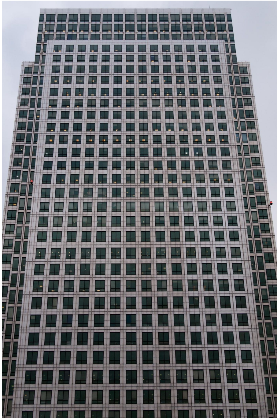
Figure 2.8: Stainless steel cladding on One Canada Square, London.
