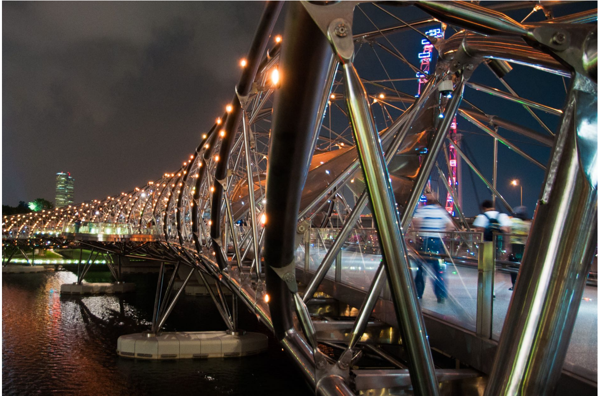
Figure 1.4: The Helix Bridge, Singapore with a stainless steel CHS truss.
