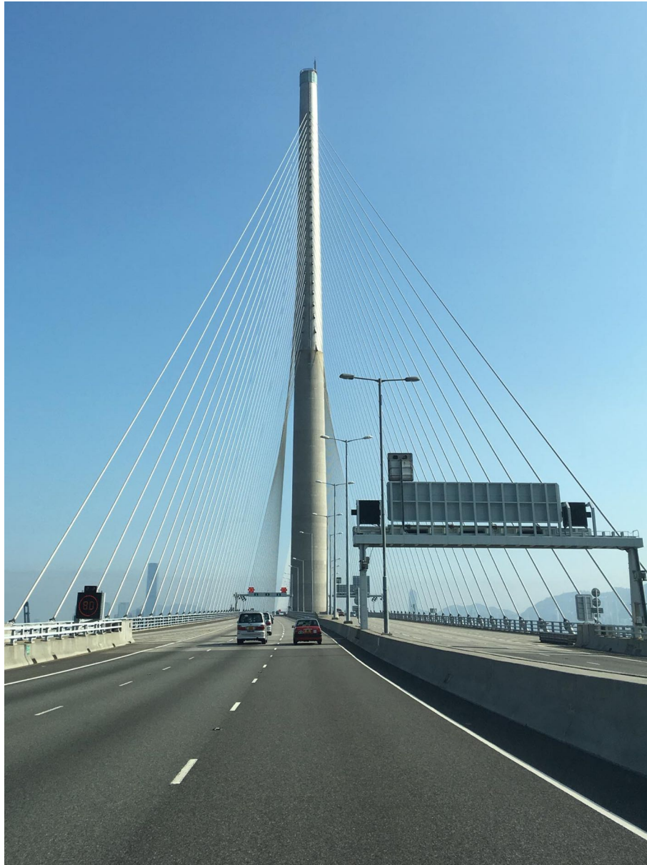
Figure 2.9: The Stonecutters Bridge, Hong Kong with a composite stainless steel skin on the upper portion of the main towers.
