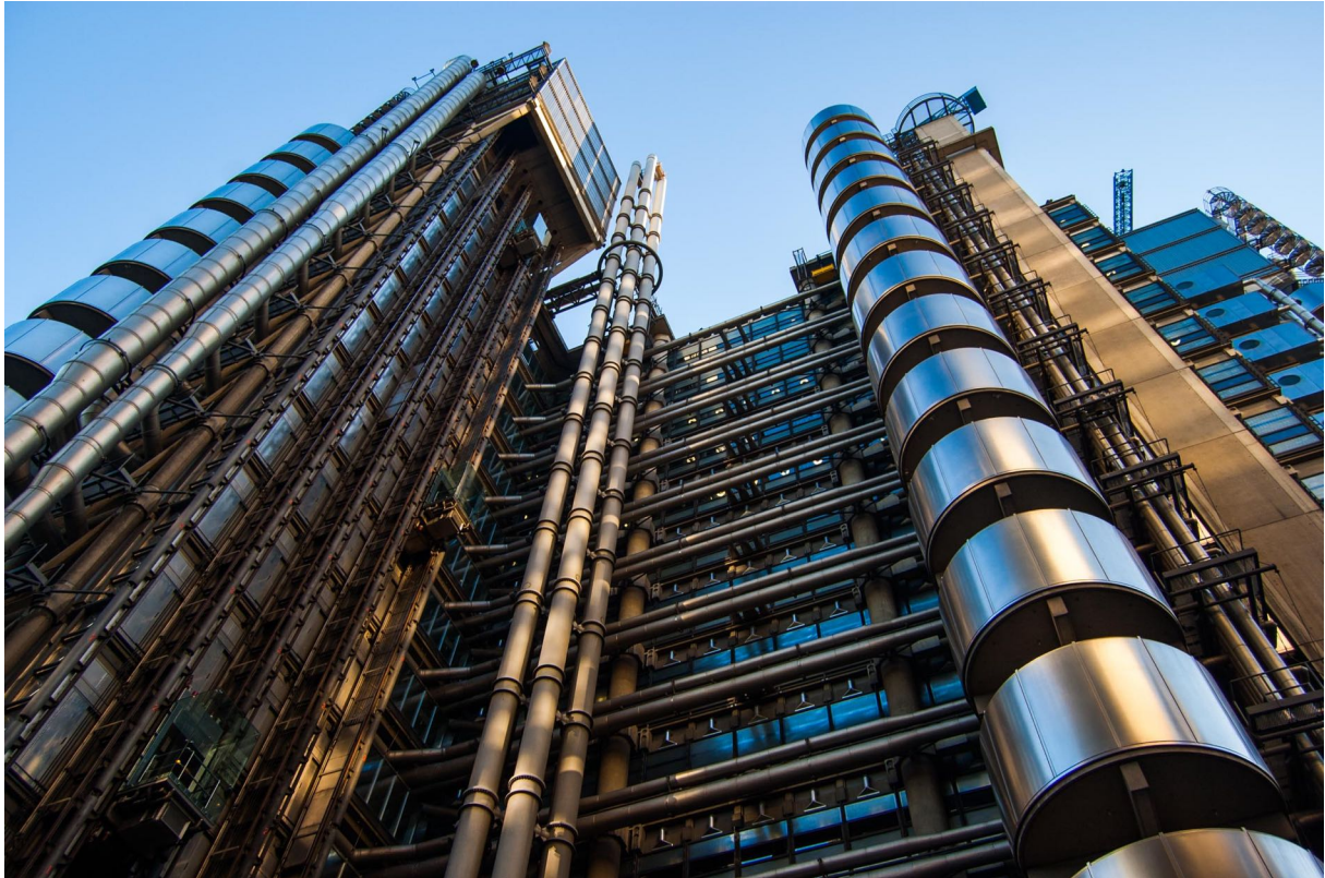
Figure 2.7: The Lloyd's Building, London with 30,000 m 2 of stainless steel cladding and pipework.
