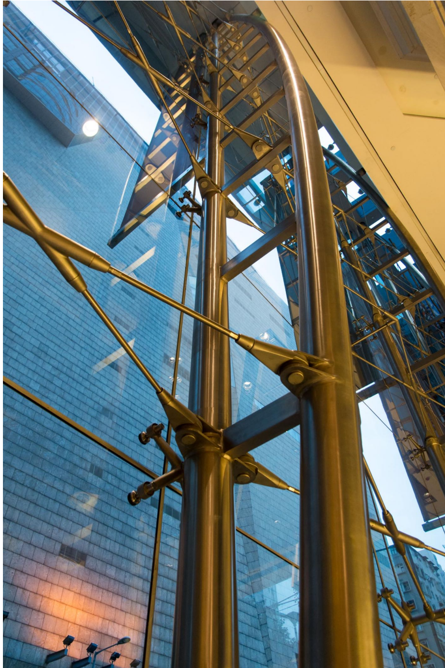
Figure 1.5: Stainless steel CHS in the entrance lobby of the Cordis Hotel, Mong Kok, Hong Kong.
