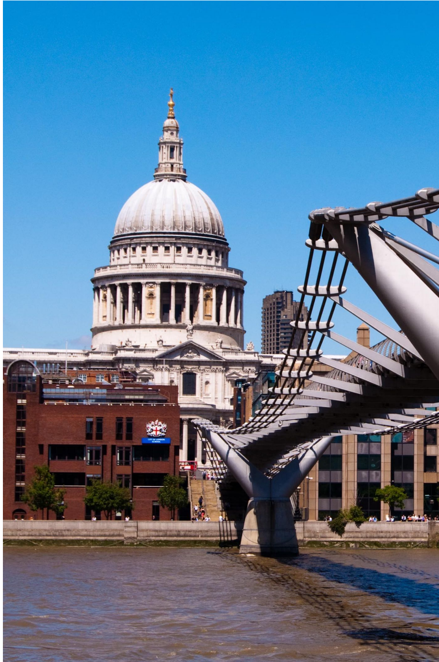
Figure 2.6: The dome of St Paul's Cathedral, London with stainless steel circumferential bands.
