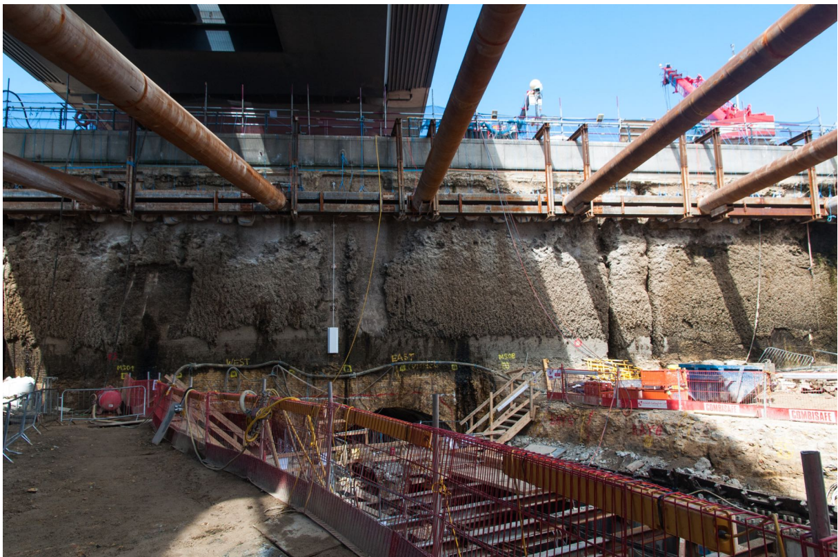
Figure 2.5: The Connaught Tunnel cofferdam, Newham, London with CHS props supporting the dock walls.
