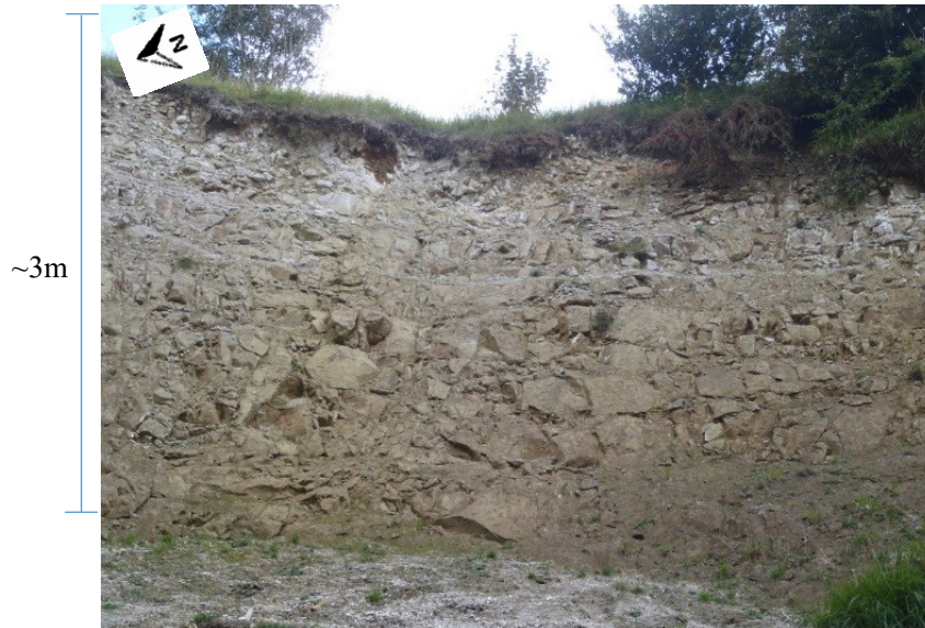
Figure 3-12: Outcrop of chalk within 1km of the Station ELSH. This shows the quality of the chalk which appears shattered in the near surface, but with increasing blockiness with depth. This is labelled as the exposure in Figure 3-10.
