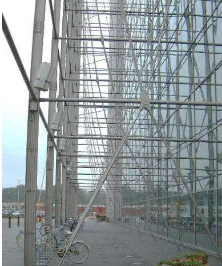
Figure 1: Sanomatalo Building, Helsinki
