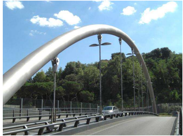
Figure 6: Road bridge near Siena
