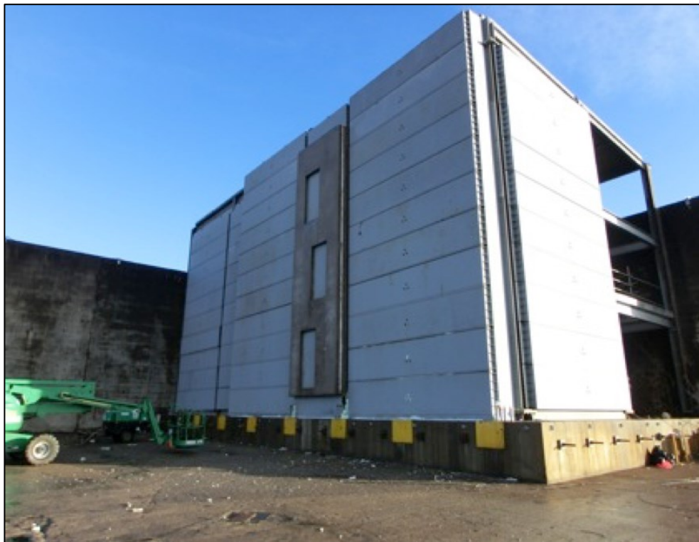
Figure 3-1 – Photograph of Large Explosion Test Facility
