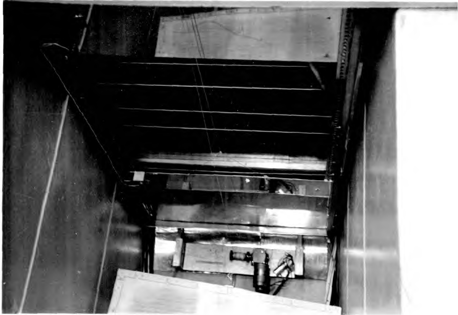
Plate 4 - View down into cave with tank removed, showing shutter in open position. Graphite extension stack and monitor counter may be seen through the window.
