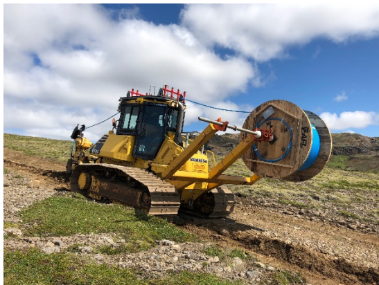
FIGURE 4: (a) Location of wells at the Hellisheidi site. HN-16 is the CO 2 injection well. The blue line is the helically wound cable deployment and the black line is the tactical cable joining the HWC to the DAS interrogator, (b), (c), (d) installation of the HWC at the Hellisheidi geothermal site.
