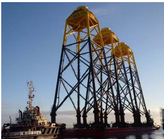
Figure 3 Photograph of three offshore wind turbine jacket structures in transit for installation at Wikingen; courtesy of Scottish Power Renewables
