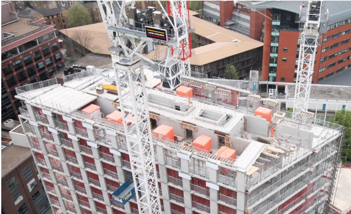
Figure 12: View of Two Fifty One during construction
