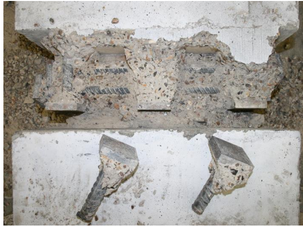
320 321 Figure 13: Failure planes after removal of headed bars
