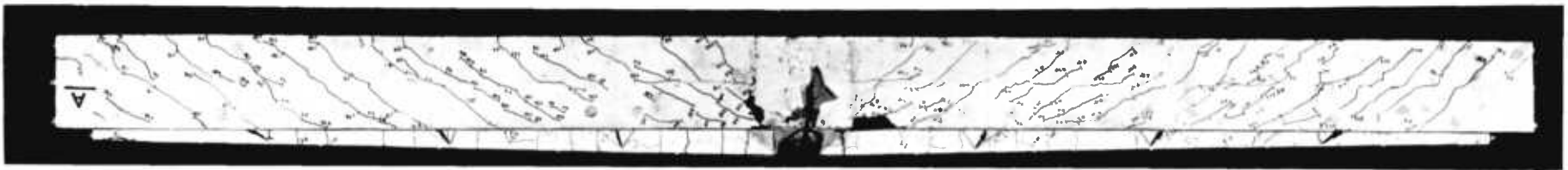
Plate 5.5 Crack Development on I-Section with Double Stirrup Reinforcement
