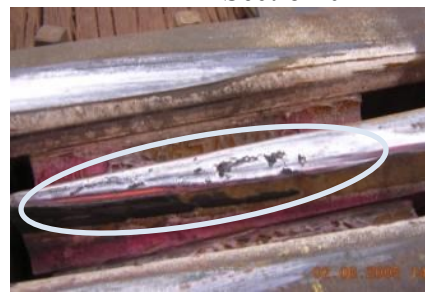
iv) Spalling / pitting – Section 4.1.4
