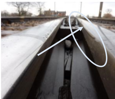
i) Plastic deformation – Section 4.1.1
