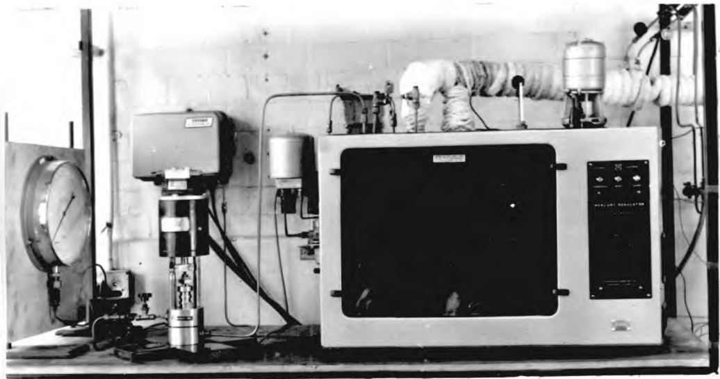
STEAM CONTROL VALVE AND SATURATOR FIG.6
