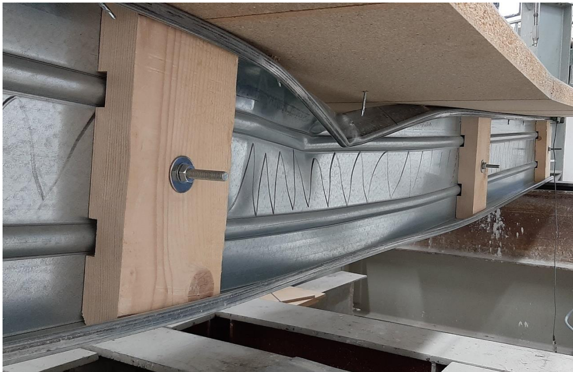
Fig. 13. Failure of specimen No. 1 – Distortional buckling within the constant moment region
