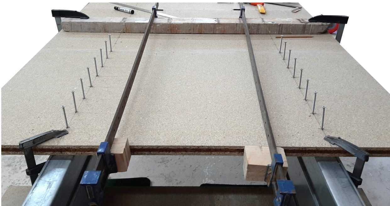
Fig. 11. Minimising gaps by clamping new board to the one previously installed
