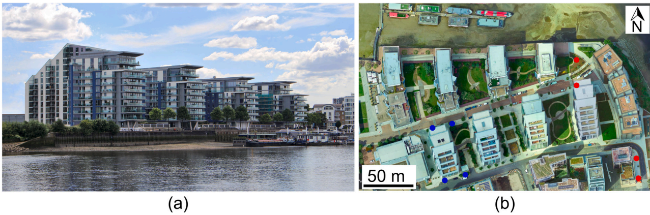
Fig. 5. (a) Photograph of Wandsworth Riverside Quarter. (b) Aerial image of the site; well locations shown by blue and red circles for cold and warm wells respectively. Source: Modified from [46].
