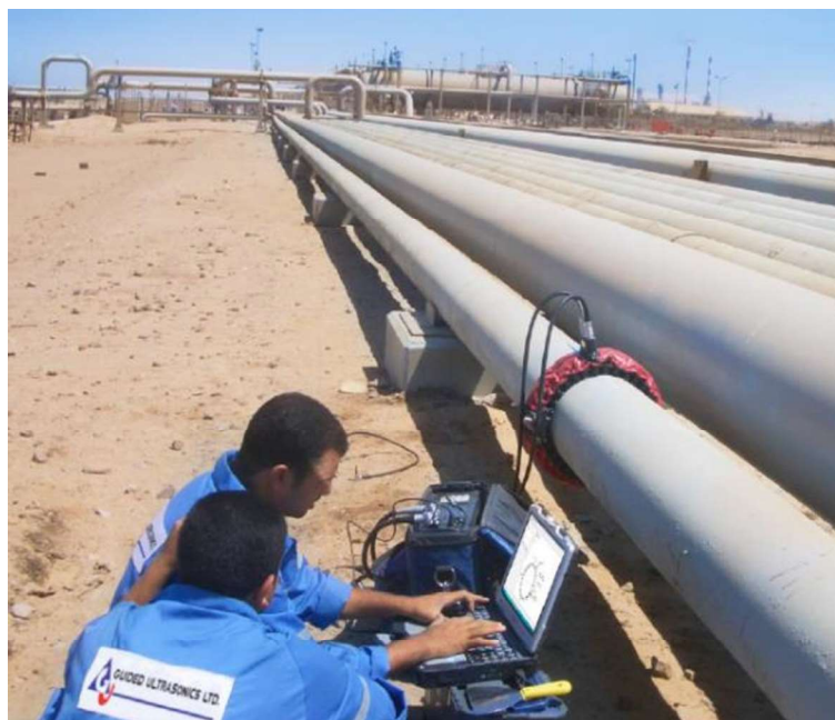
Figure 1.1: A snapshot of pipe GWT inspection of industrial pipelines. [1]
